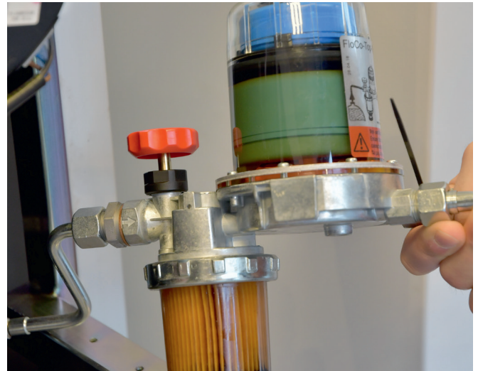
Heating oil filter and degasser
